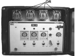
Fig. 6. A static (electronic) protection device with large-output electromechanical relays of industrial type, placed in separate cell (OR – output relays)
